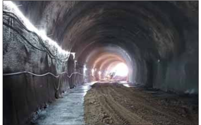
Obr. 2 Vyražený tunel v plném profilu Fig. 2 Excavated tunnel in its full profile
