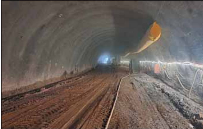
Obr. 1 Vyražená kalota tunelu Fig. 1 Excavated top heading of the tunnel
