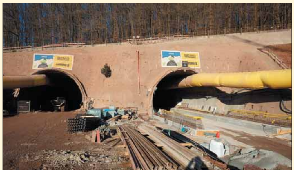
Obr. 1 Portál VTT a ZTT (pohled zprava) tunelu Holstein Fig. 1 ETT and WTT portal (view from the right) of the Holstein tunnel
