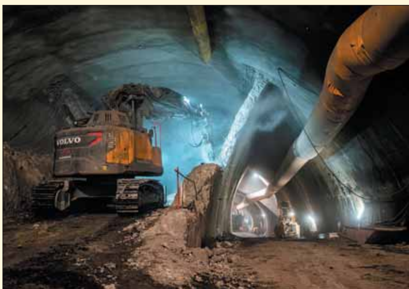
Obr. 1 Momentka z ražeb kaloty stanice Pankrác Fig. 1 Snapshot from the excavation of the top heading at the Pankrác station
