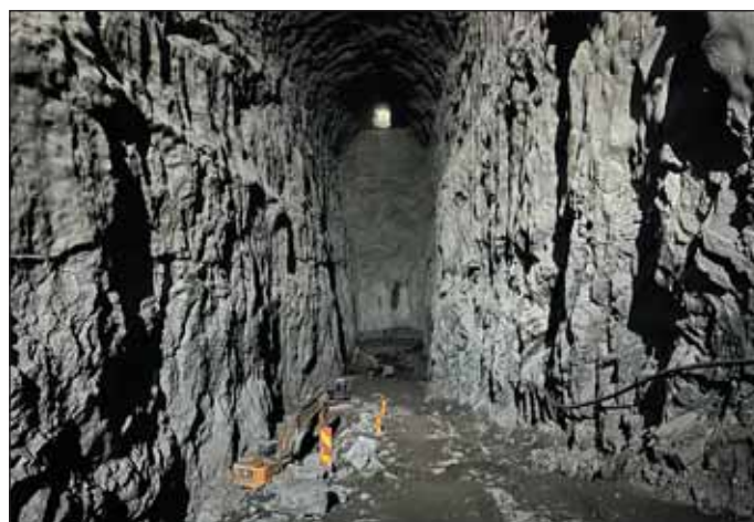
Obr. 6 Pohled do téměř vyražené kaverny 23 Fig. 6 View into the almost excavated No. 23 cavern
