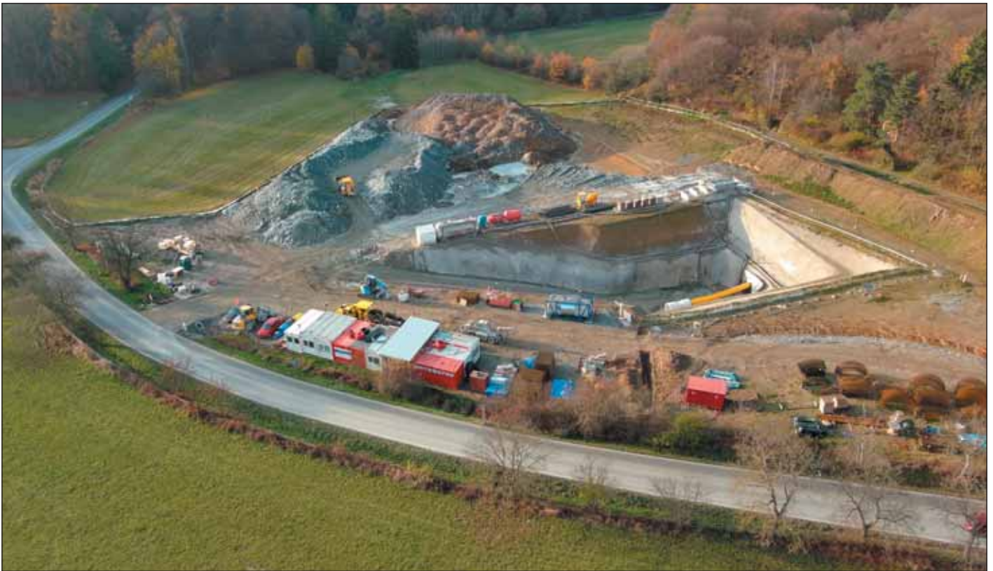
Obr. 3 Portálová jáma u křižovatky silnic II/104 a III/1042 Fig. 3 Portal pit by the intersection of roads II/104 and III/1042
