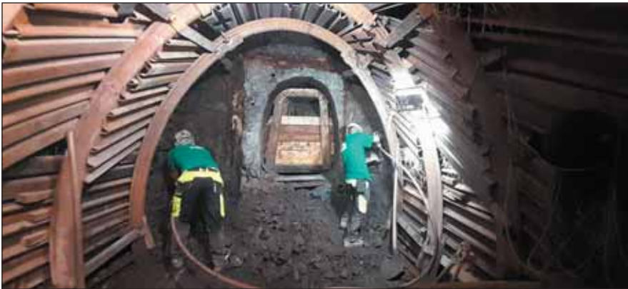
Obr. 3 Prerážba štoly X. Fig. 3 Re-excavation of the X. gallery
