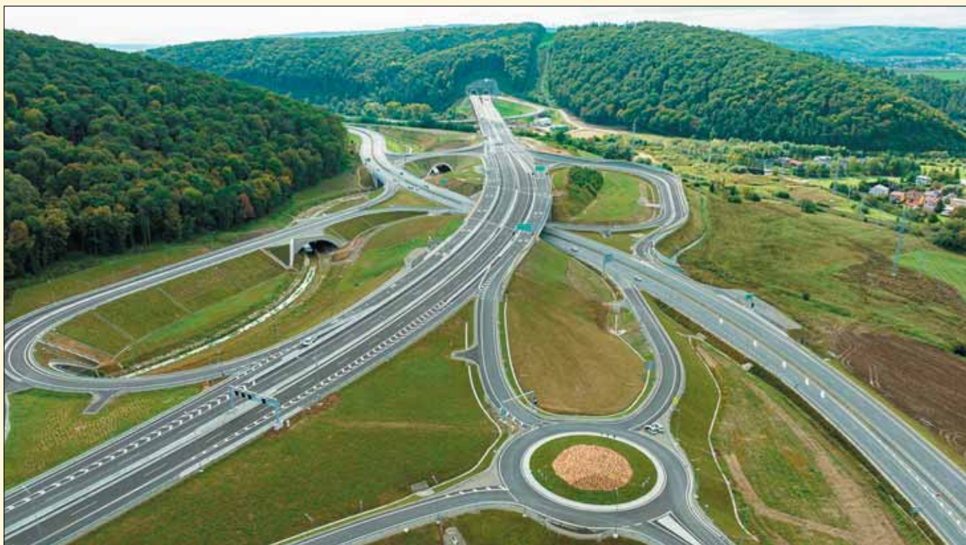
Obr. 3 Mimoúrovňová križovatka pred severným portálom tunela Bikoš Fig. 3 Grade separated intersection before the northern portal of the Bikoš tunnel
