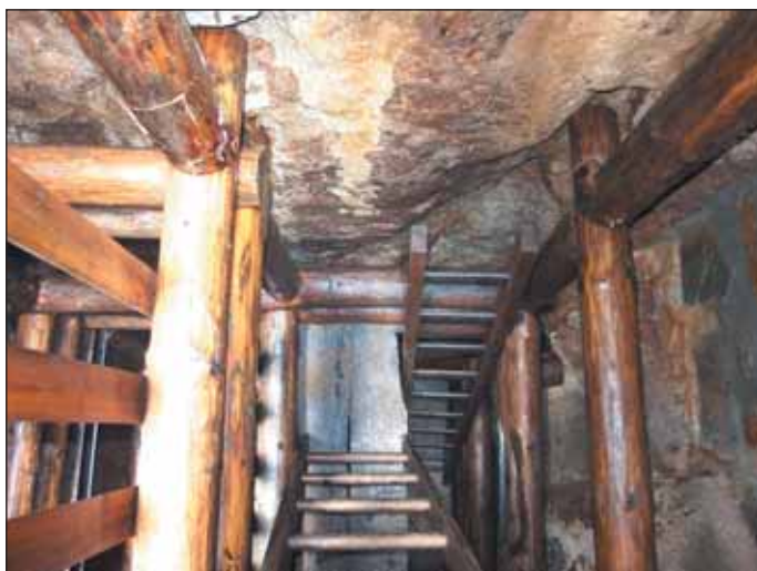
Obr. 7 Stará šachta u silnice po vystrojení v duchu 16. století Fig. 7 An old shaft by the road after being supported by the methods of the 16 th century
