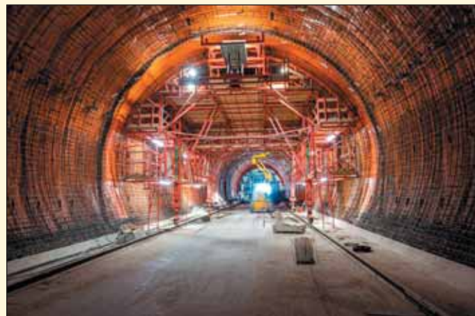
Obr. 2 Realizace armatury jižního tunelu Fig. 2 Placement of reinforcement in the southern tunnel tube
