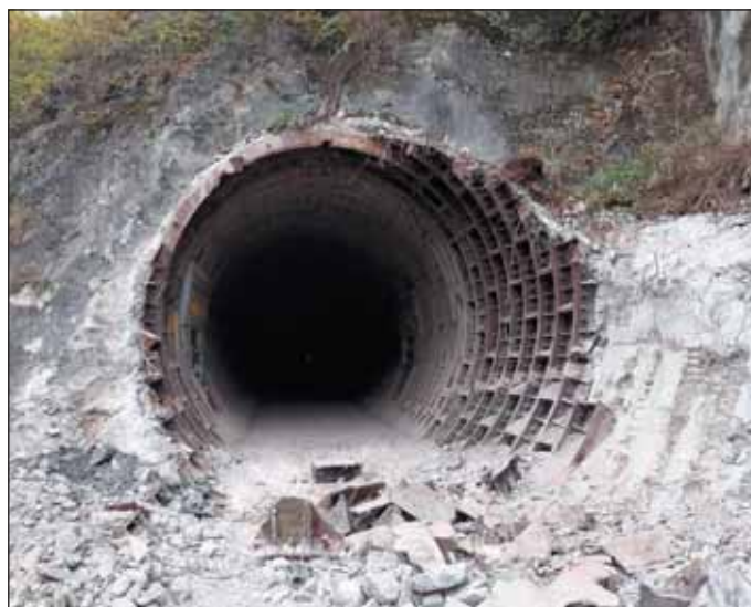
Obr. 2 Litinové a železobetonové tubingy, portál P1 (Adamov) Fig. 2 Cast iron and reinforced concrete lining segments, P1 portal (Adamov)
