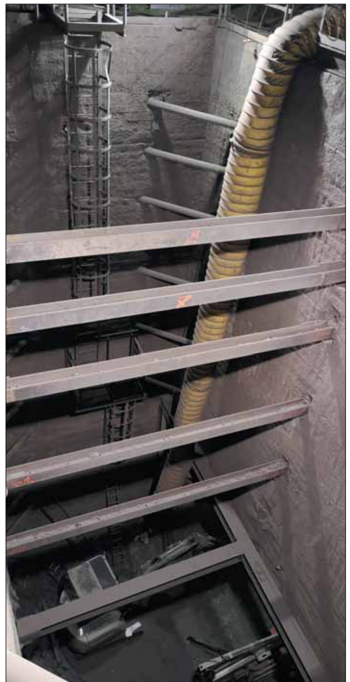
Obr. 6 Hloubená šachta Š2.1 Fig. 6 Excavated shaft Š2.1
