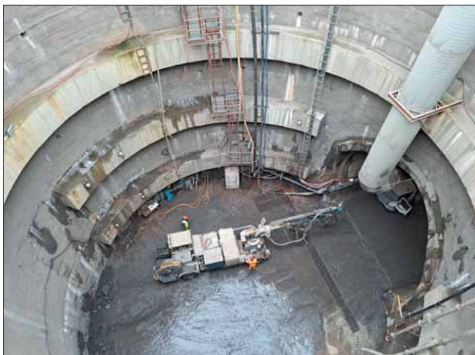
Obr. 2 Šachta na staveništi PAD1b Fig. 2 Shaft at the construction site PAD1b
