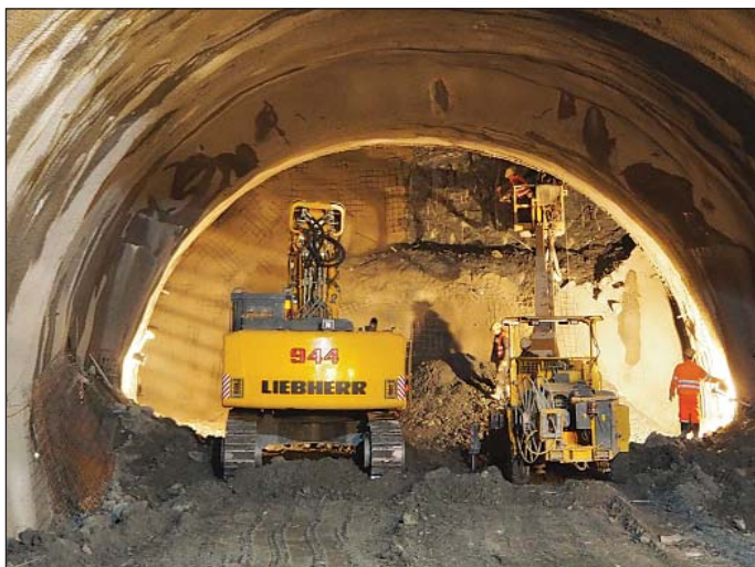
Obr. 3 Razenie tunela Fig. 3 Tunnel excavation
