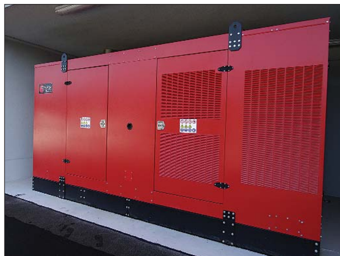
Obr. 4 Dieselagregát pre tunel Poľana Fig. 4 Diesel generating set for the Poľana tunnel
