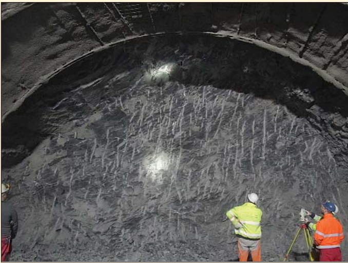
Obr. 9 Tunel Diel, čelba tvorená ílovcami Fig. 9 Diel tunnel, excavation face formed by claystone
