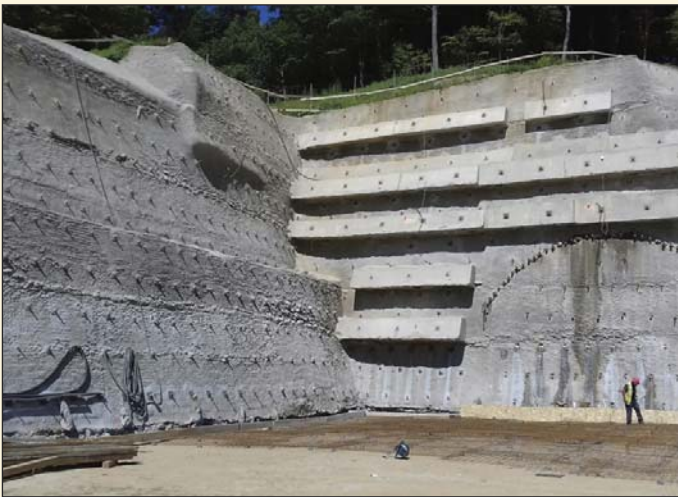
Obr. 3 Tunel Prešov Fig. 3 Prešov tunnel
