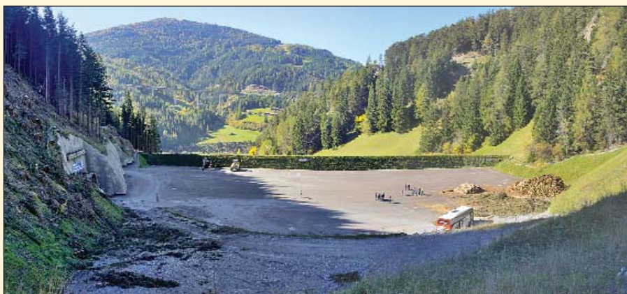
Obr. Deponie Padastertal pro 7,7 mil. m 3 rubaniny Fig. Padastertal stockpile for 7.7M m 3 of muck
