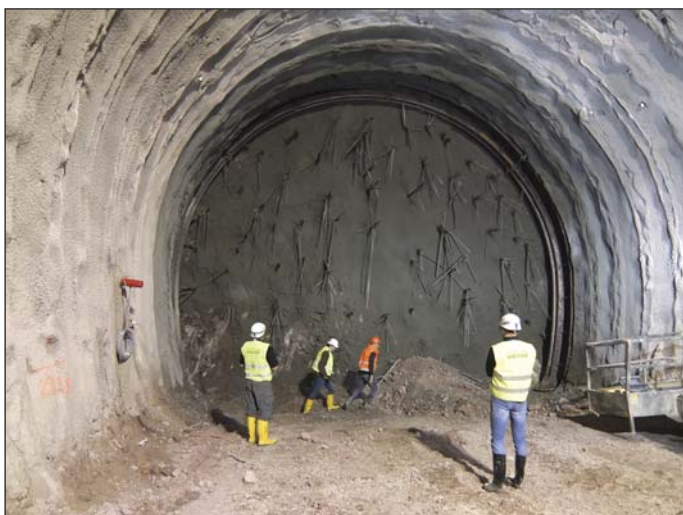
Obr. 5 Konsolidačné opatrenia v čelbe tunela vo vstrojovacej triede B0/3 Fig. 5 Consolidation measures at the tunnel heading through excavation support class B0/3
