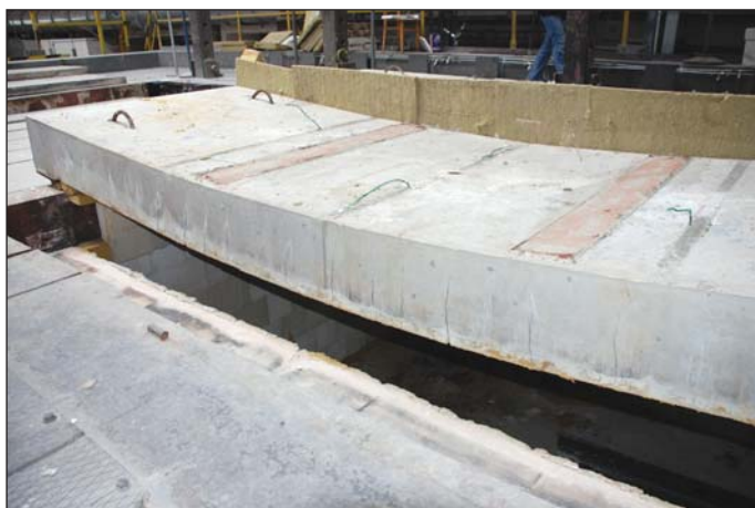
Obr. 7 Vzorek po zkoušce s viditelnou velikostí deformace Fig. 7 A sample after testing, showing a visible magnitude of deformation
