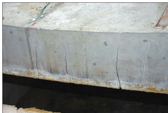
Obr. 8 Detail velikostí trhlín Fig. 8 A detail of the magnitude of cracks
