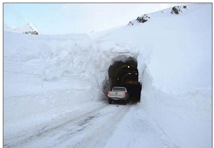
Obr. 1 Pohled na portál tunelu Oddskardgöng Fig. 1 View of the Oddskardgöng tunnel portal
