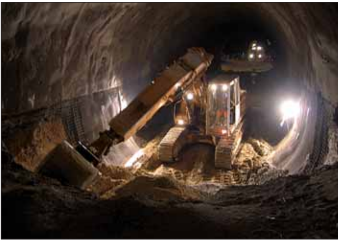
Obr. 6 Výlom lavice a dna tunela Fig. 6 Bench and invert excavation
