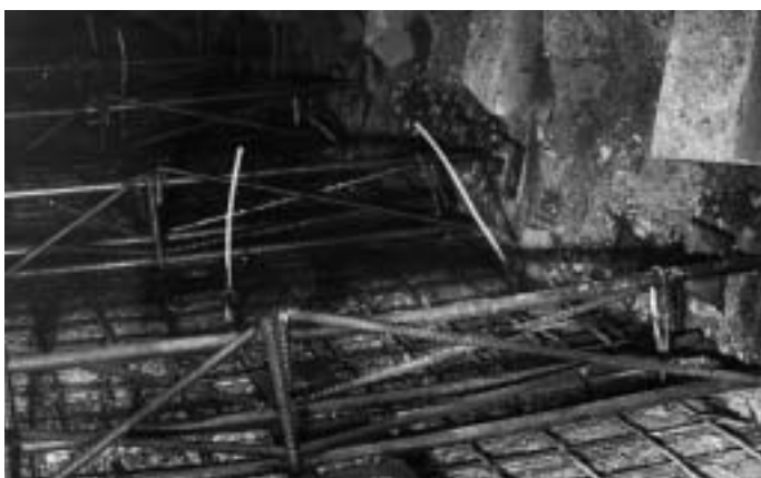
Obr. 4 Sychrovský tunel Fig. 4 The Sychrov tunnel
