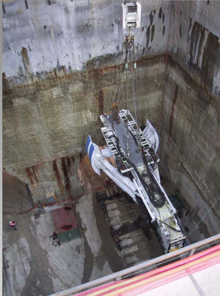
Lowering TBM Down the Shaft Epping to Chatswood Rail Link
