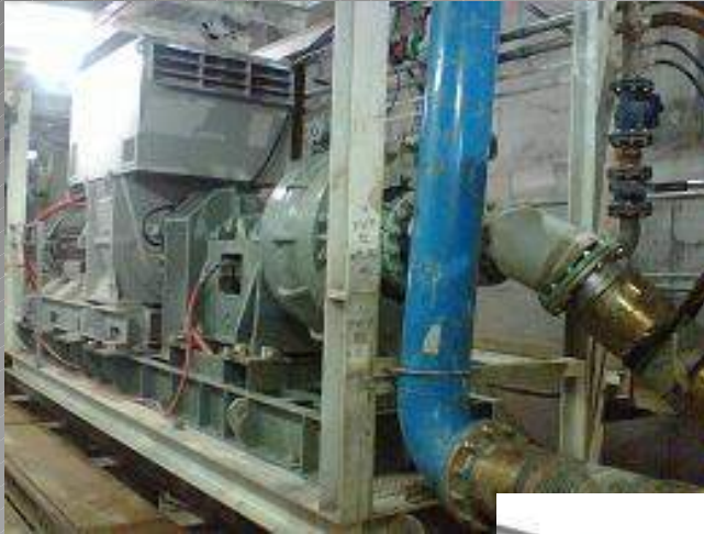
Slurry Discharging Pump
