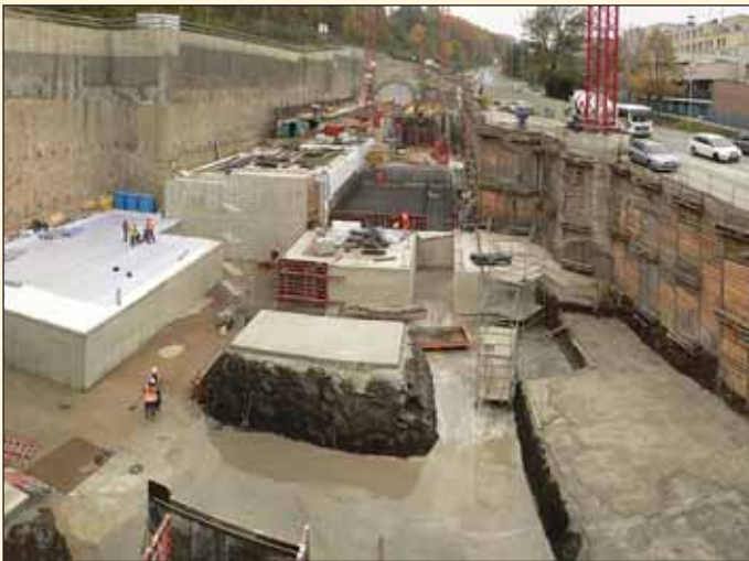
Z výstavby stanice Motol na trase V.A From the construction of the Motol station on V.A line
