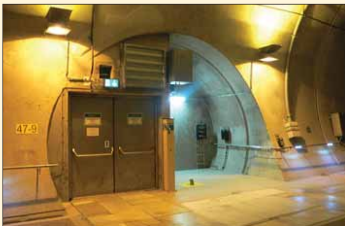
Obr. 3 Úniková cesta – propojka mezi tunely Wienerwald Fig. 3 Escape route – a cross passage between the Wienerwald tunnel tubes
