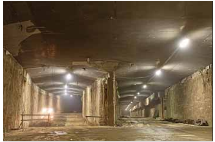
Obr. 6 Rozplet vjezdové rampy 2 a jižního tunelu u Hradčanské Fig. 6 Bifurcation of the exit ramp No. 2 and the southern tunnel tube near Hradčanská station
