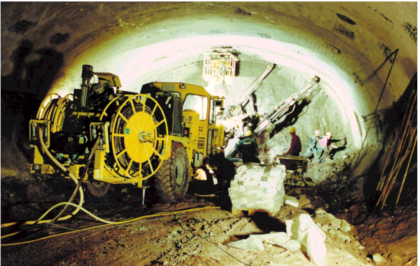
Obr. 5 Budovanie SN kotiev v tuneli Gäubahn Fig. 5 The installation of SN anchors in the Gäubahn tunnel
