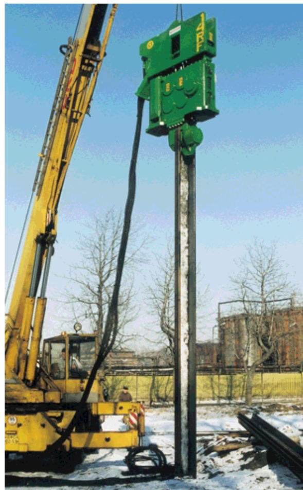
Obr. 3 Beranidlo ICE 14 RF Fig. 3 Pile-driver ICE 14 RF
