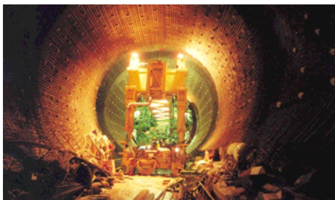
Obr. 4 Debniaci voz pred presunom do nového bloku betonáže Fig. 4 The movable formwork before moving into new concrete placement block
