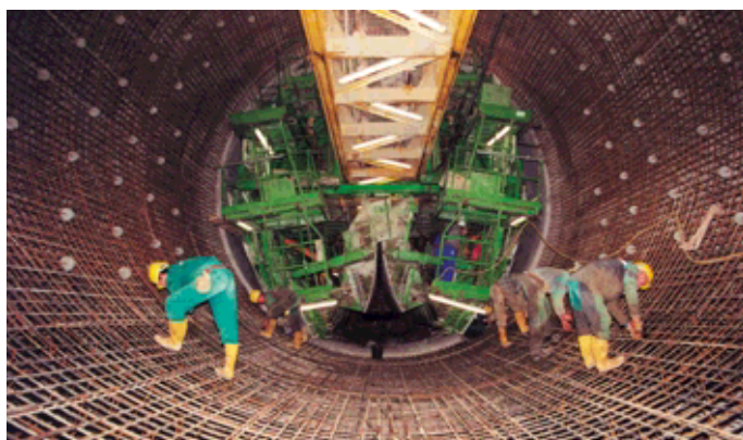
Obr. 5 Uzavretie celokruhovej armatúry pred presunutím debniaceho voza Fig. 5 Closing of the reinforcement circle before moving the formwork
