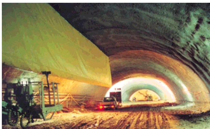
Obr. 7 Kalota tunela Dölszchen Fig. 7 The Dölszchen tunnel top heading
