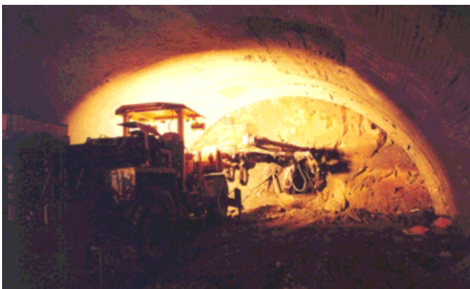
Obr. 2 Vrtné práce v kalote tunela v úseku s predrazenou prieskumnou štôľňou Fig. 2 Drilling in the top heading, in the section with the pre-excavated exploration gallery
