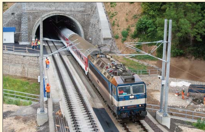
Obr. 2 Severný portál tunela (foto Juraj Michalka) Obr. 2 Northern portal of the tunnel (photo courtesy of Juraj Michalko)
