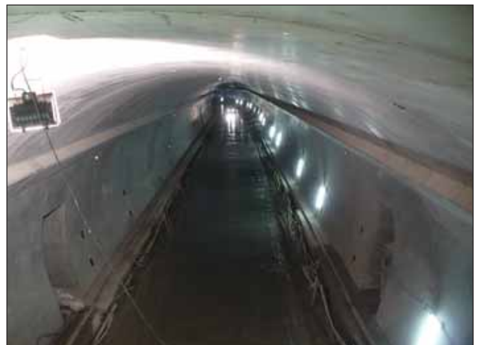
Obr. 12 Pohled dovnitř tunelu z mezistropu Fig. 12 View inside the tunnel from the intermediate deck
