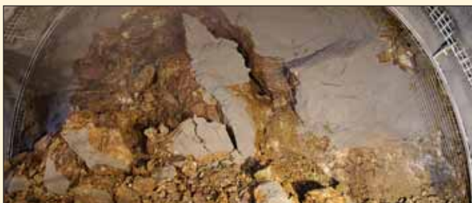
Obr. 4 Nestabilita čelby Fig. 4 Instability of the face
