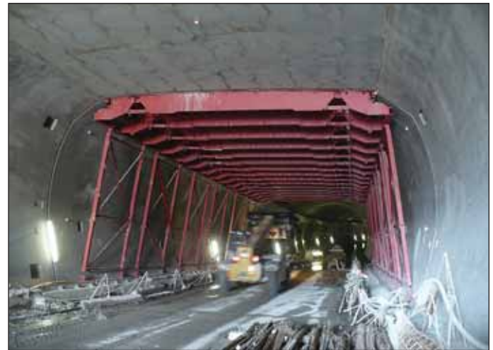
Obr. 14 Pohled na bednicí stoly mezistropu Fig. 14 View of intermediate deck-forming tables
