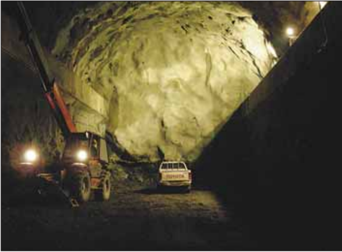
Obr. 5 Kaverna podzemnej strojovne so zabetónovanou žeriavovou dráhou Fig. 5 The cavern for the underground turbine hall with the concrete crane track casting completed
