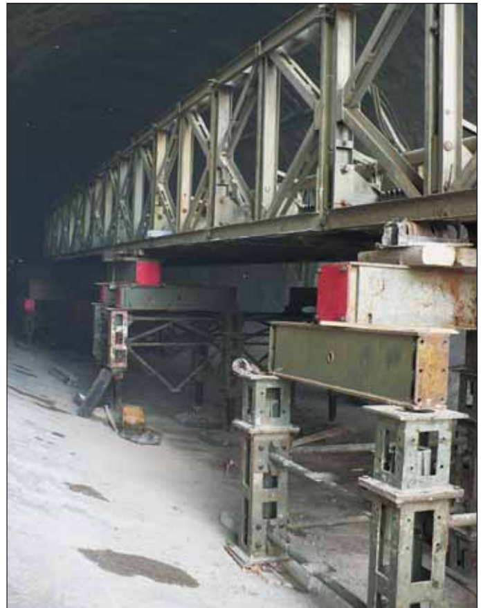
Obr. 17 Ženíjní most v tunelu Fig. 17 Steel military bridge in the tunnel
