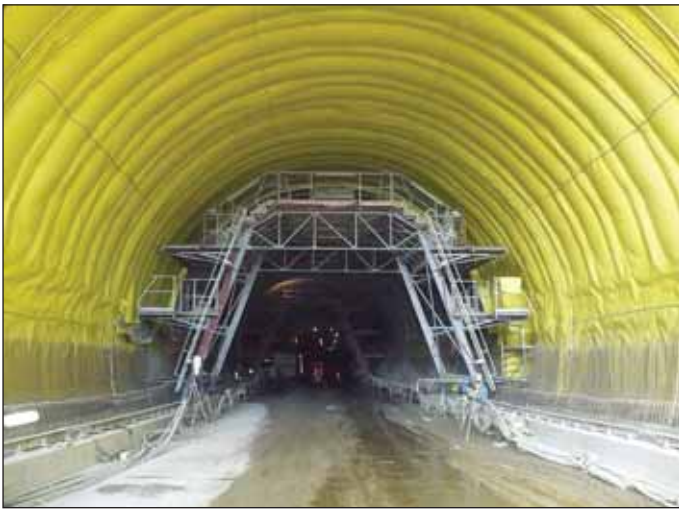
Obr. 11 Pohled na izolační platformu a provedenou izolaci klenby v tunelu Fig. 11 View of a waterproofing installation platform and waterproofing completed in the tunnel vault
