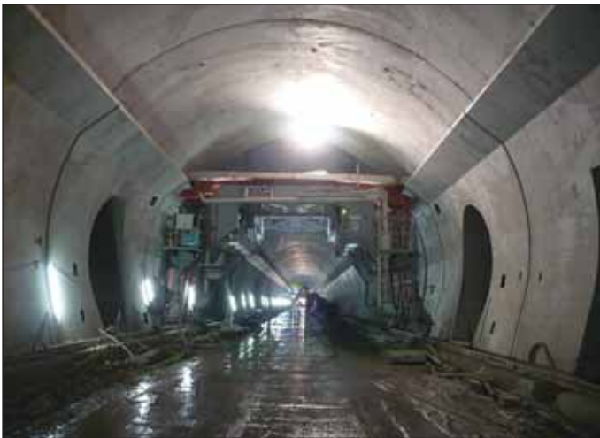
Obr. 13 Pohled na obslužný vůz pro bednicí stoly mezistropu Fig. 13 View of the service vehicle for the intermediate deck-forming tables
