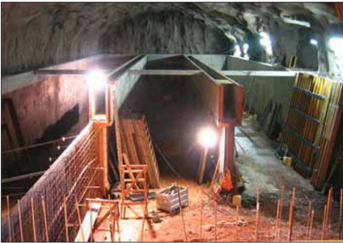
Obr. 6 Prepojovacia stredová žľabová stena – sedimentácia – nitrifikácia Fig. 6 An interconnecting central trough-wall between the sedimentation and nitrification section
