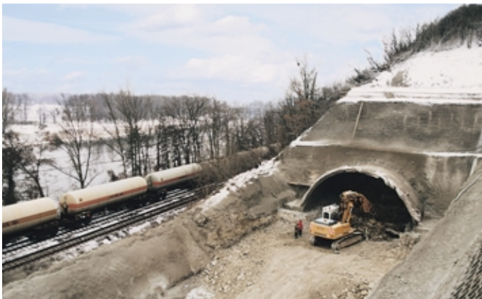
Obr. 2 V lednu 2001 byly vyraženy bagrem Liebherr 932 první metry kaloty Fig. 2 In January 2001 the first metres of the top heading were excavated
