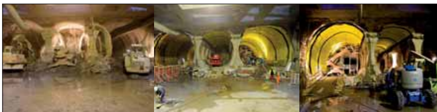
Obr. 10 Ražená stanice Gellert Fig. 10 Gellert mined section
