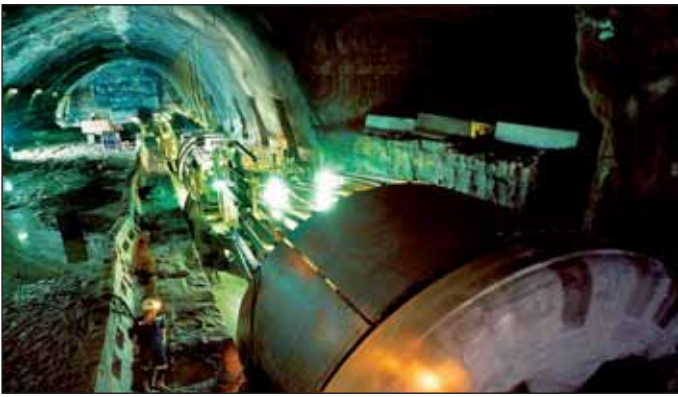
Obr. 4 Ražby stroji TBM ve stanici Macquarie Park Fig. 4 TBM bores through Macquarie Park Station
