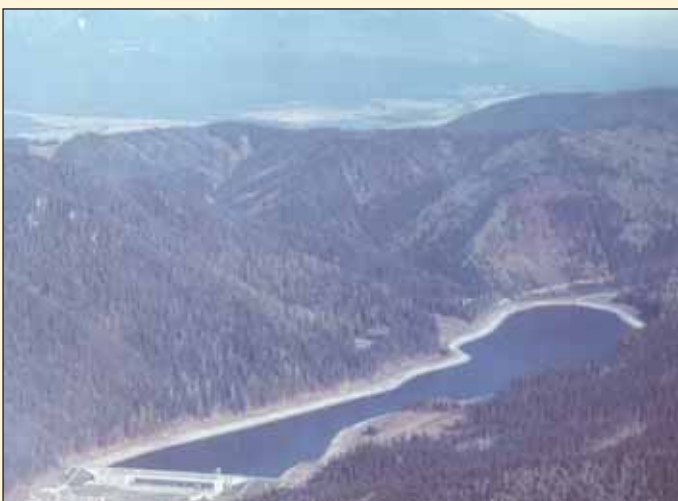
Obr. 1 Pohľad na elektrárň s dolnou nádržou Fig. 1 A view of the power plant with the downstream reservoir
