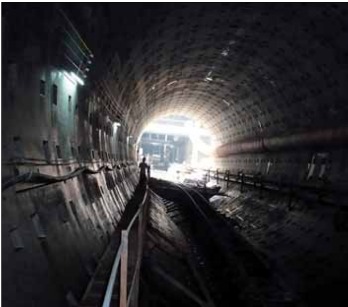
Obr. 5 Pohled do šachty z dokončeného tunelu Fig. 5 View to shaft from the completed tunnel
