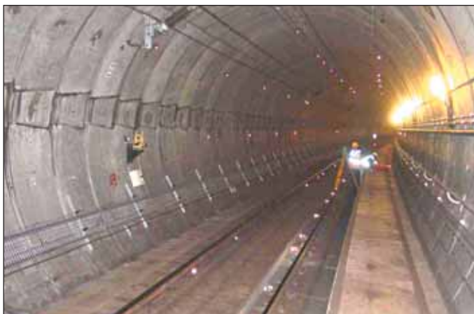
Obr. 12 Monitoring tunelu trati Heathrow Express (automatický teodolit a terče) Fig. 12 Monitoring of Heathrow Express tunnel (robotic theodolite and targets)
