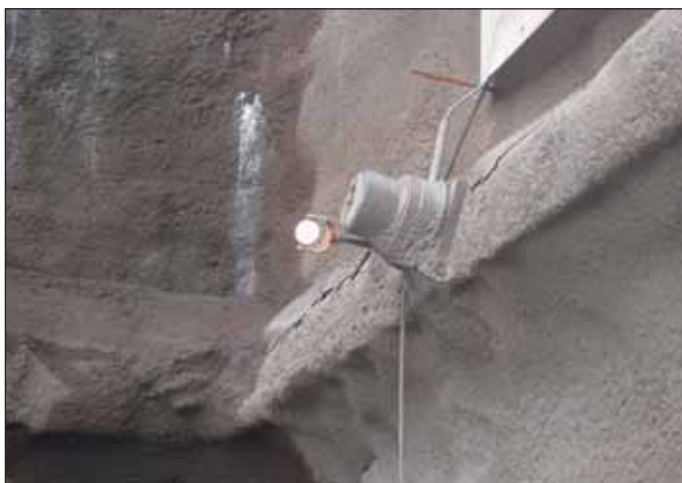
Obr. 5 Detail hlavy kotvy osazené dynamometrem a geodetickým bodem Fig. 5 Detail of an anchor head with a tensionmeter and survey point installed
