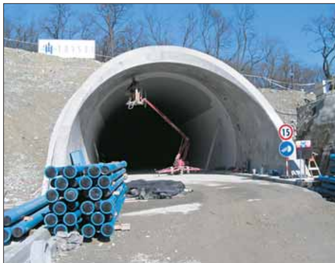
Obr. 3 Južný portál tunela Fig. 3 Southern portal of the tunnel
