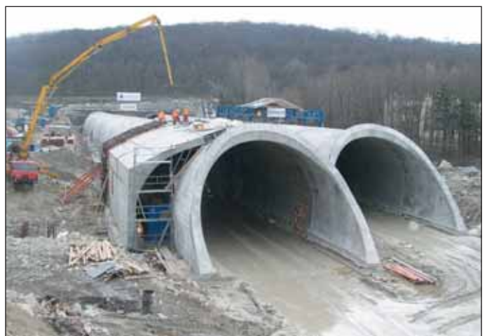
Obr. 3 Hĺbené úseky tunela Sitina na severnom portáli Fig. 3 Cut-and-cover sections of the Sitina tunnels at the north portal
