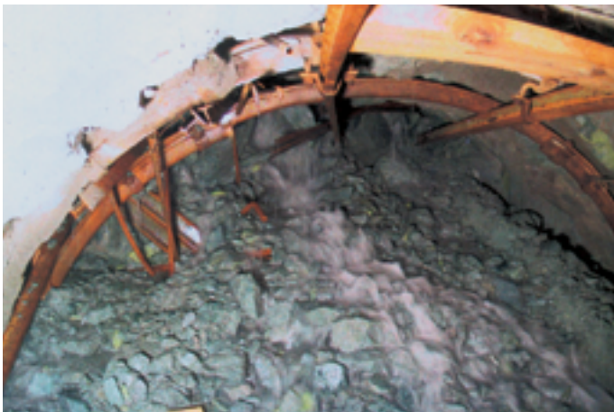
Obr. 10 Závall spôsobený sufóznym účinkom tlakovej vody v tektonickej poruche na ZP Fig. 10 The collapse due to solid transport caused by pressure water in the tectonic disturbance at the WP
