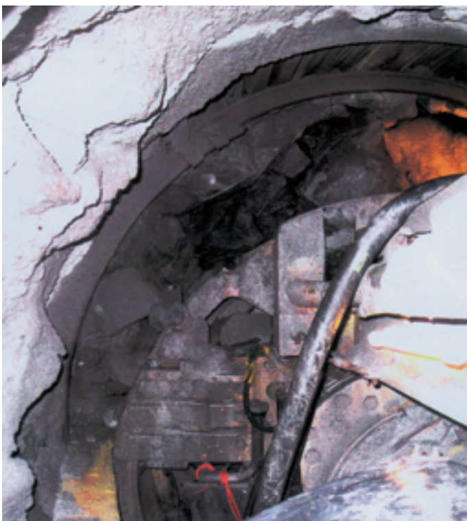
Obr. 12 Nevhodná blokovitost horniny pred raziacim strojom Fig. 12 Unfavourable blockiness of rock ahead of the TBM
