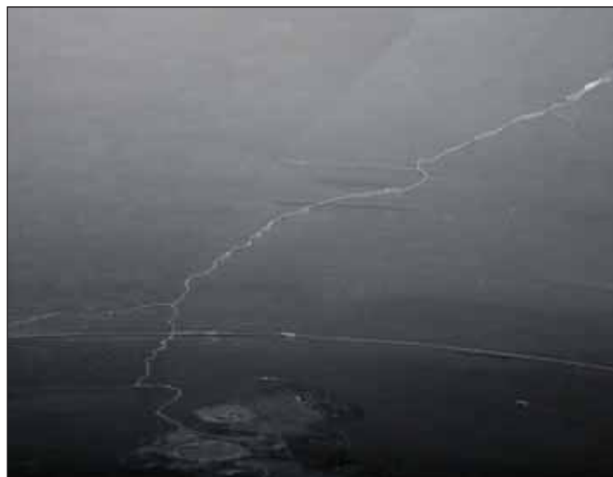
Obr. 10 Trhliny ve vrcholu klenby tunelu Roppen Fig. 10 Crack in the crown of Roppen tunnel
