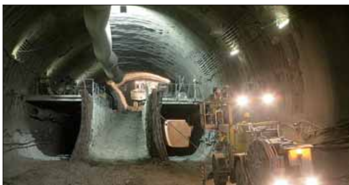
Obr. 3 Ražba kaloty tunelu Fig. 3 Tunnel top heading excavation
