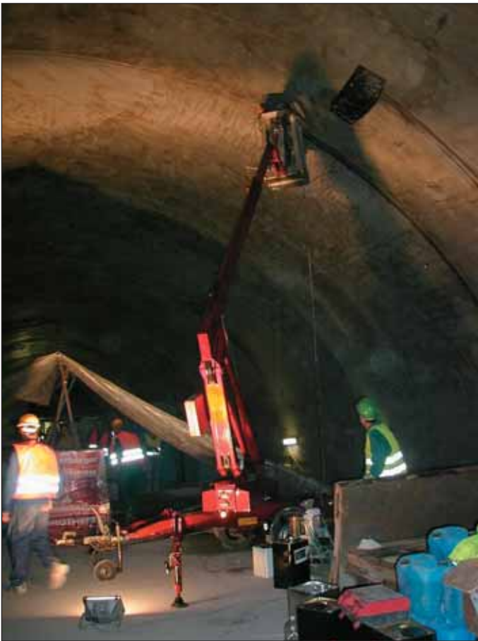
Obr. 2 Metro IVC1 – injektáž spáry v klenbě stanice Kobylisy Fig. 2 Metro IVC1 – grout injection into a joint in the vault of the Kobylisy station
