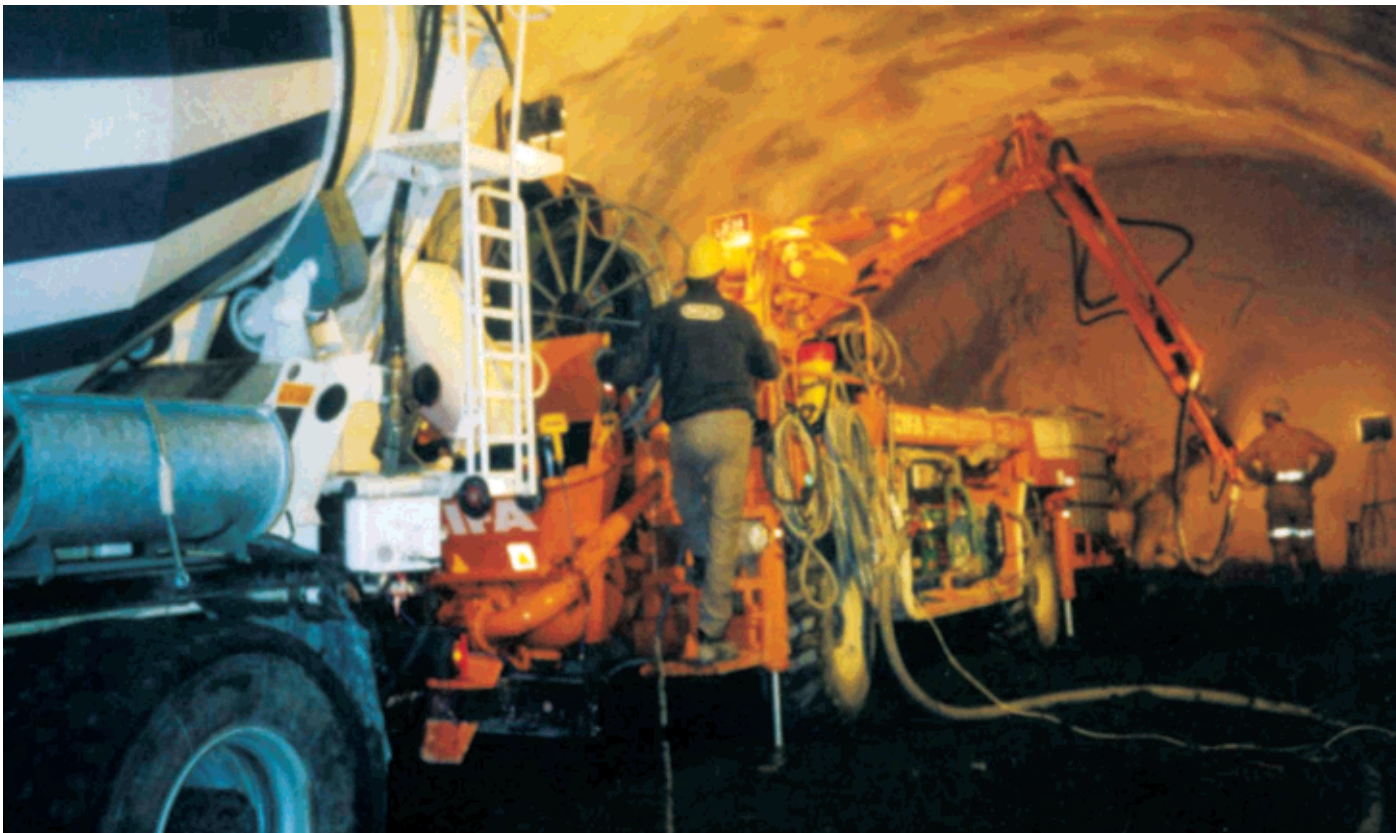
Obr. 1 Vystrojovanie tunela Fig. 1 Supporting of the tunnel
