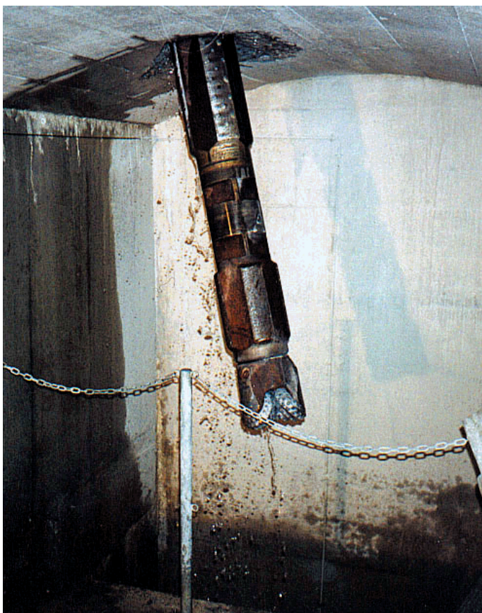
Obr. 3 Pronik pilotního vrtu do „toskomory“ Fig. 3 Pilot bore penetration into the “toss-chamber”
