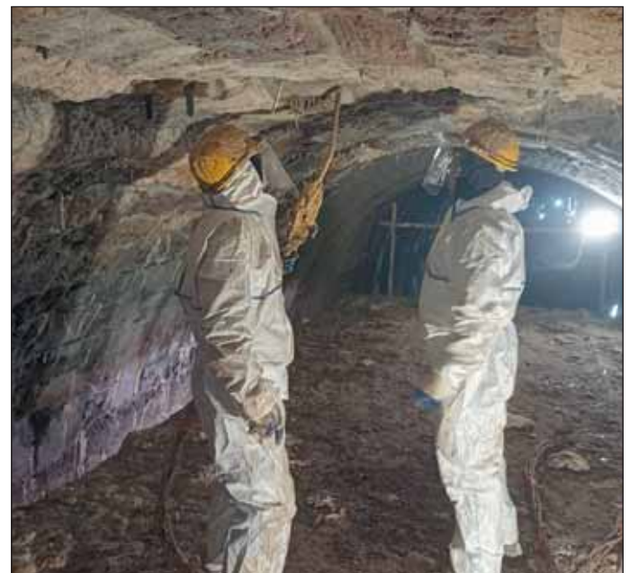
Obr. 7 Reinjektáž v klenbe tunela Fig. 7 Reinjection in the tunnel vault
