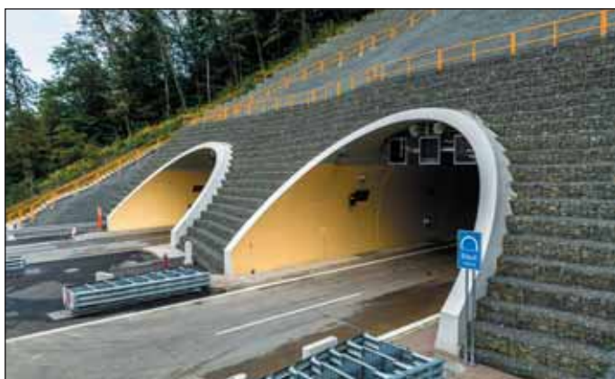
Obr. 5 Severný portál tunela Fig. 5 Northern portal of the tunnel
