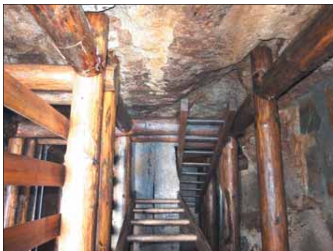
Obr. 7 Stará šachta u silnice po vystrojení v duchu 16. století Fig. 7 An old shaft by the road after being supported by the methods of the 16 th century
