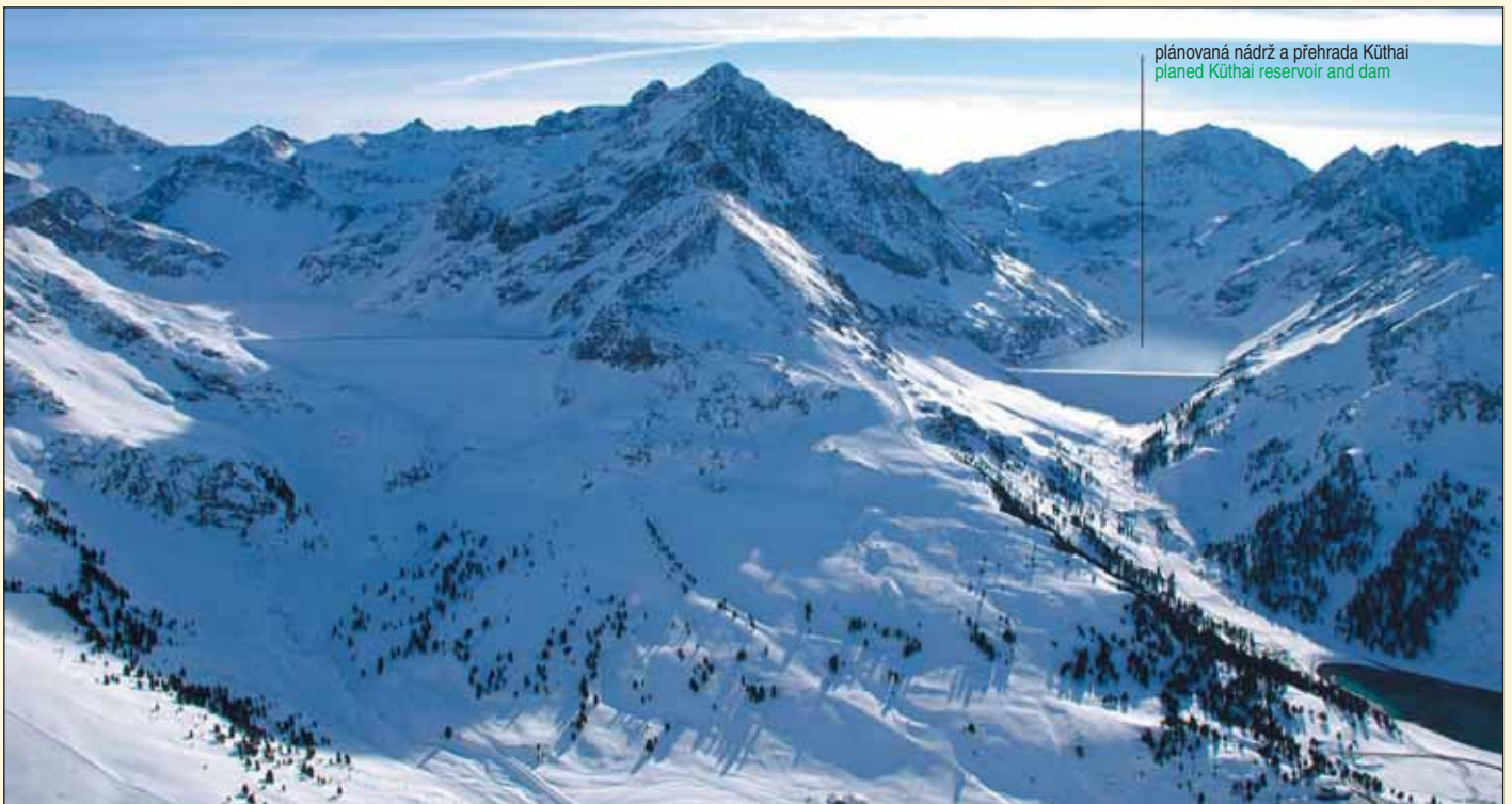
Obr. 1 Celkový pohled na PVE Kühltal Fig. 1 Overall view of the pumped storage power plant Kühltal
