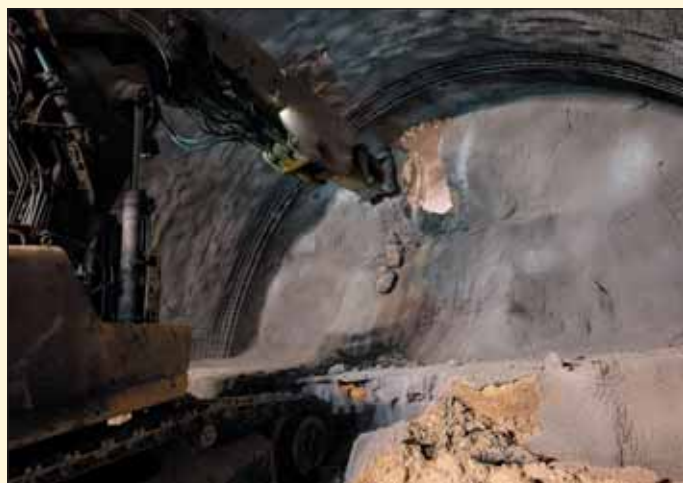
Obr. 2 Okamžik strojní prorážky severního tubusu tunelu Fig. 2 Moment of mechanical breakthrough of the northern tube of the tunnel
