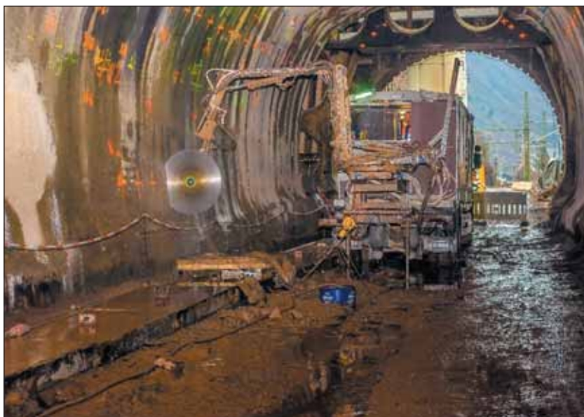
Obr. 5 Prerezávanie ostenia kotúčovou diamantovou pilou prispôsobenou na použitie v tuneli Fig. 5 Cutting through the lining with diamond disc cutter accommodated to the use in tunnel
