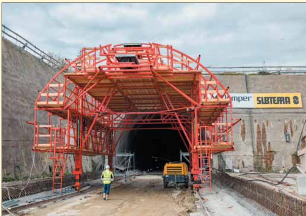
Obr. 1 Vůz na montáž ocelové armatury Fig. 1 Movable scaffold for assembly of steel reinforcement
