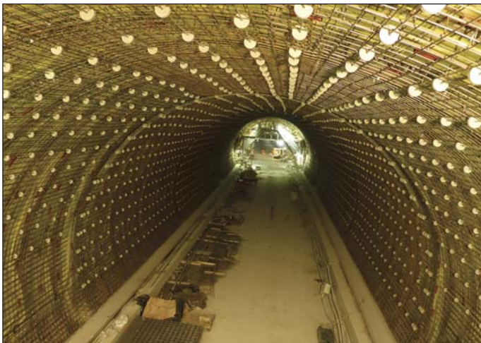
Obr. 1 Armatúra hornej klenby Fig. 1 Upper vault concrete reinforcement
