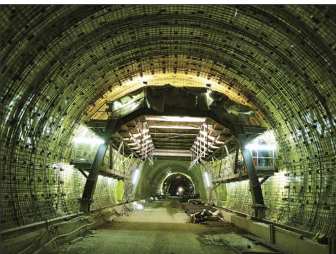
Obr. 5 Montáž armatúry hornej klenby Fig. 5 Installation of concrete reinforcement of the upper vault
