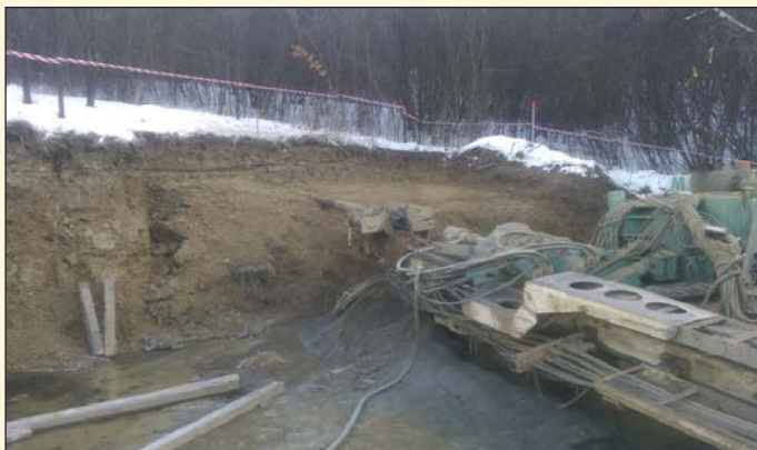
Obr. 3 Odvodňovacie vrty na západnom portáli tunela Diel Fig. 3 Drainage boreholes at the western portal of the Diel tunnel
