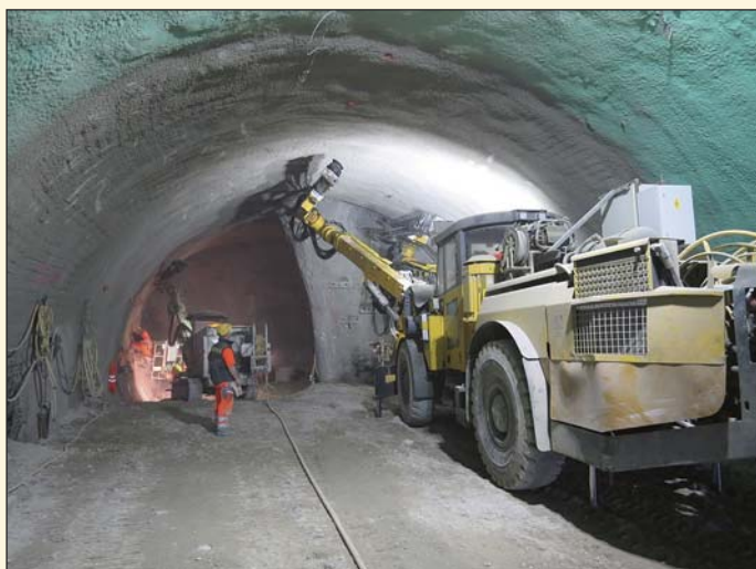
Obr. 1 Tunel Karl-Friedrich-Strasse v Karlsruhe Fig. 1 Karl-Friedrich-Strasse Tunnel in Karlsruhe
