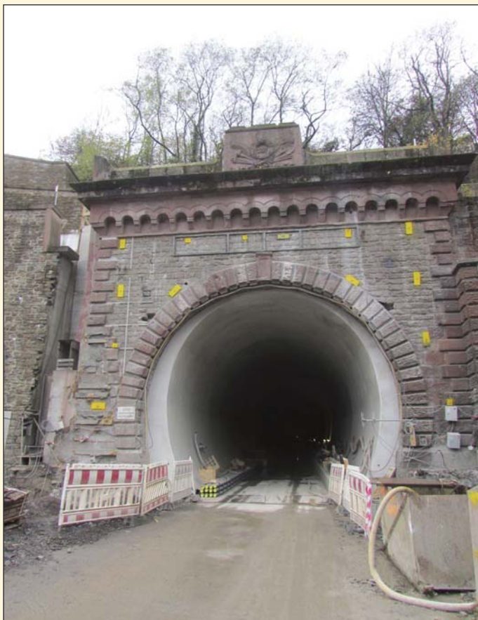
Obr. 3 Portál v Cochemu – tunel AKWT Fig. 3 Portal in Cochem – the AKWT tunnel
