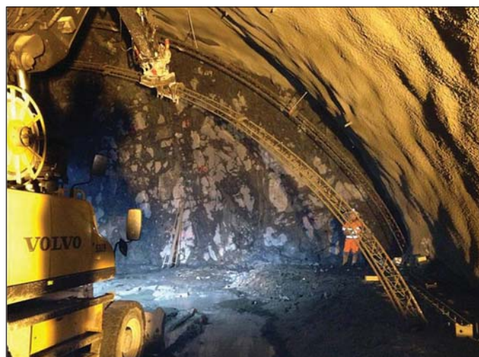
Obr. 9 Priehradové nosníky počas montáže v kalote Fig. 9 Lattice girders during the course of the assembly in the top heading
