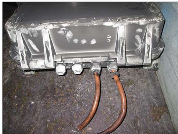
Obr. 11 Odmontované svítidlo zasažené požárem Fig. 11 Detached luminary affected by fire
