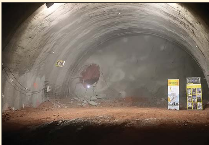
Obr. 2 Prorážka tunelu Bancarevo Fig. 2 Breakthrough of the tunnel Bancarevo
