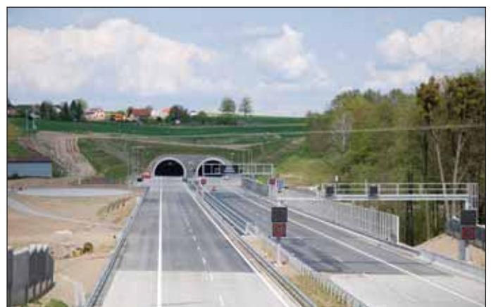
Obr. 13 Pohled na vjezd do tunelu (brněnský portál) (foto Pechman) Fig. 13 View of the tunnel entrance (the Brno portal) (photo Pechman)
