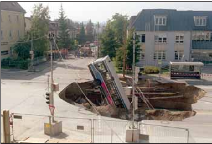
Obr. 17 Autobus zapadlý do krátera po havárii tunelu v Mnichově Fig. 17 A coach fallen to a crater due to a tunnel collapse in Munich
