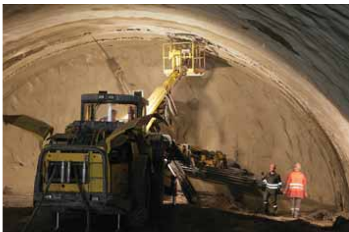
Obr. 3 Ražba kaloty STT tunelu Brusnice Fig. 3 Brusnice NTT top heading excavation
