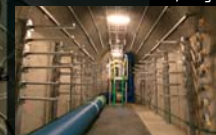
Underground Utility Tunnel Wenceslas Square - Line C, Prague
