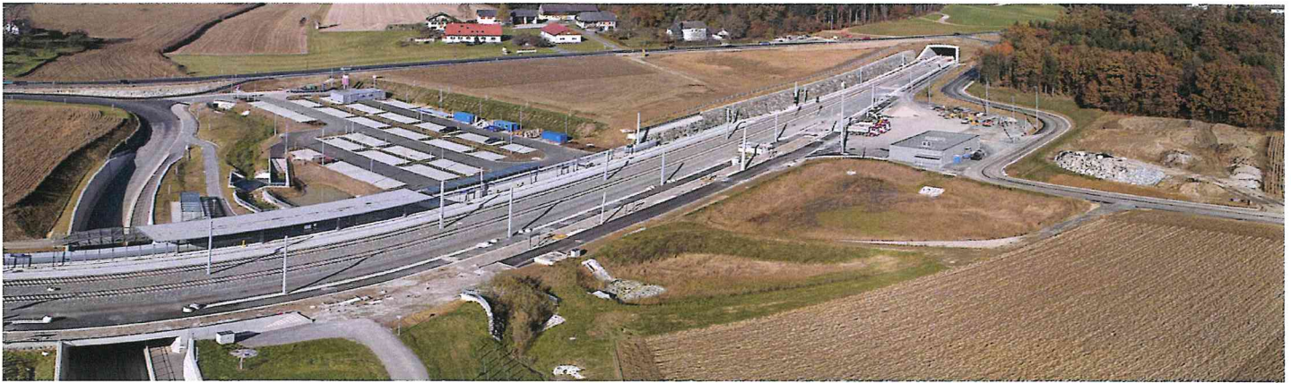
View of the new railway station at Hengsberg and the entrance to the Hengsberg Tunnel
