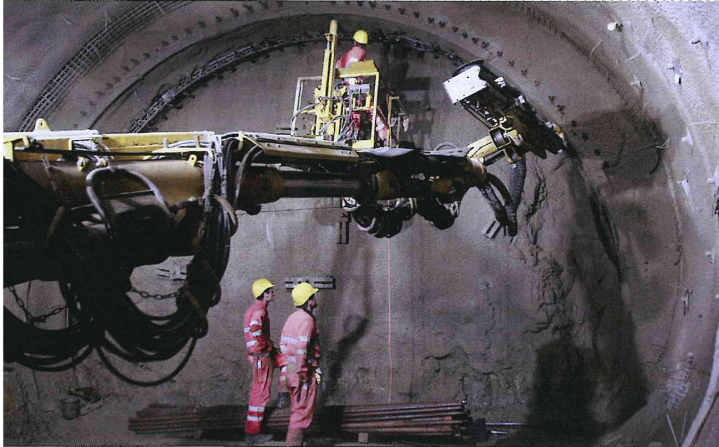
Advance tunnelling work in the Koralmbahn tunnel
