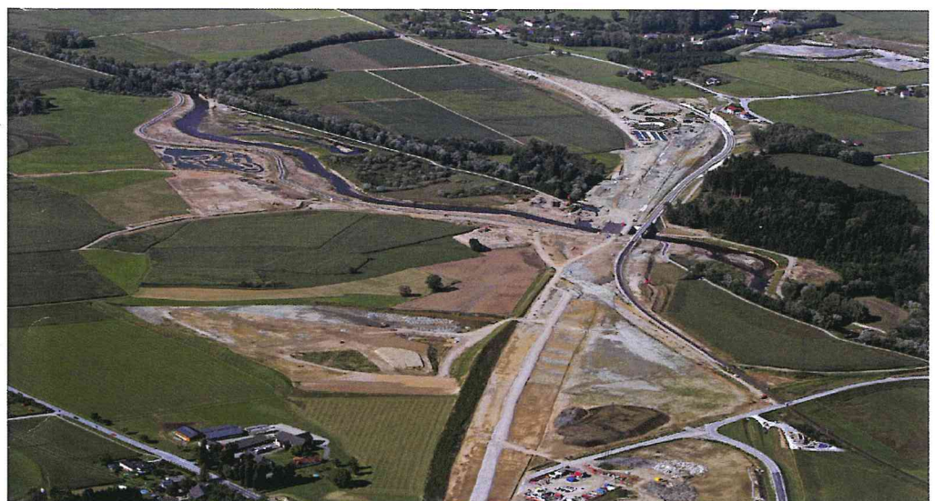
Aerial view of construction work in the Lavanttal
