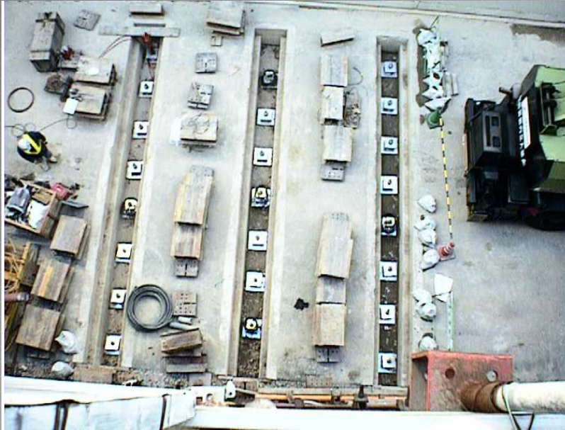
Bearing plates and anchors on the surface
