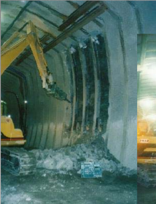
Removing steel support
