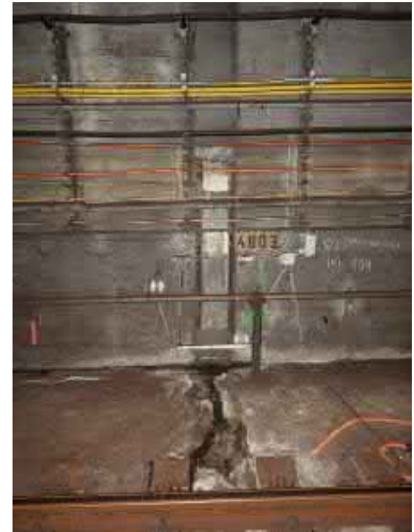
ASD dilatometry v metru C
