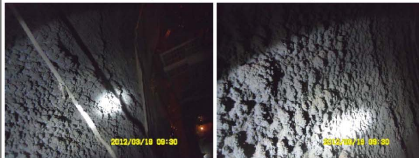
Fig. 1, 2: No right quality of primary lining close to geo textile (on both sides)
