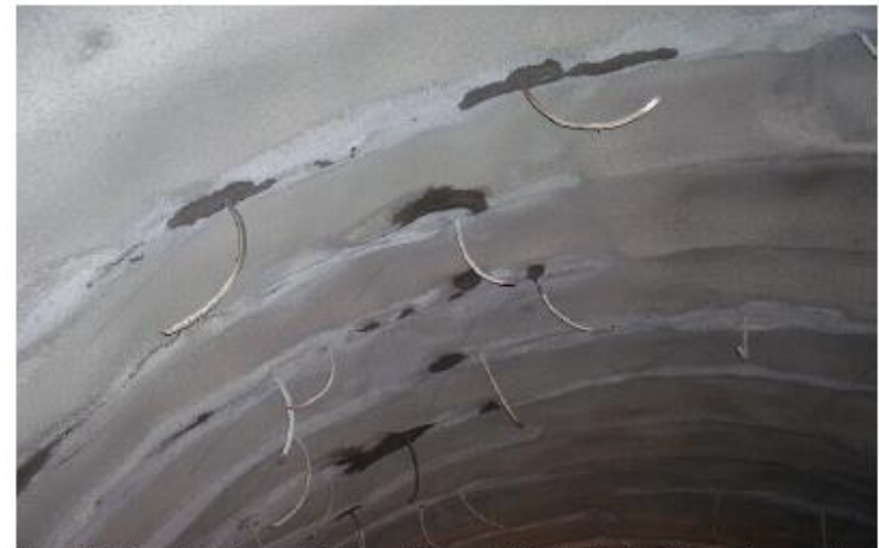
Figure 7: Photo of drainage with 10 mm diameter drillholes fitted with jet-packers and hoses, prior to the application of MASTERSEAL ® 345
